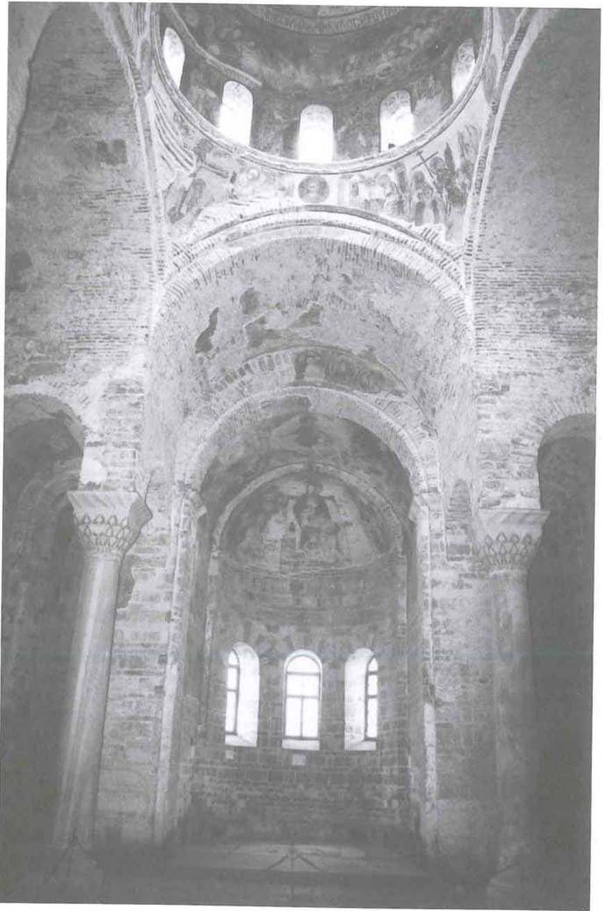
16 The main apse and dome of Hagia Sophia. The interior is very tall and light
